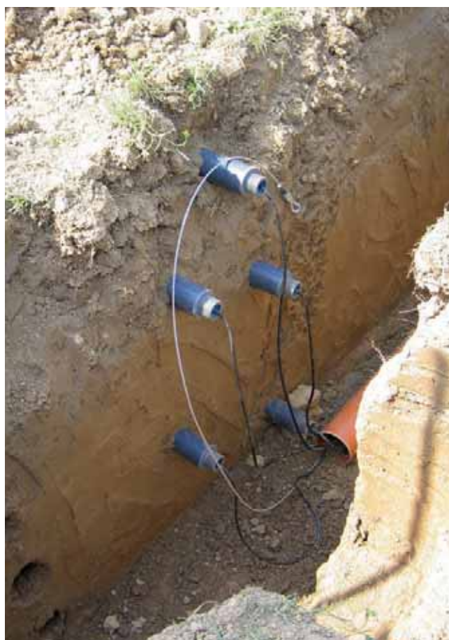
Example of the installation of PICO64 in an undisturbed subsoil
